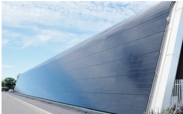
The photovoltaic wall at the OpTic Technium building in St Asaph
